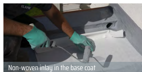
Application of base coat
